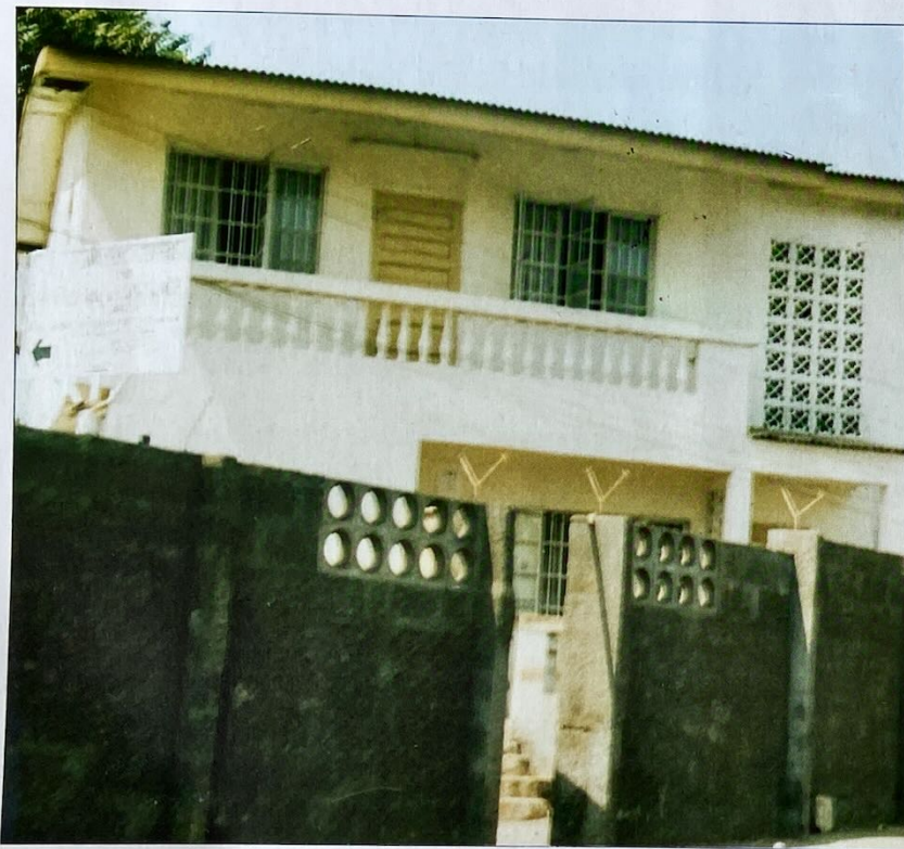
The front elevation of the Freetown office
